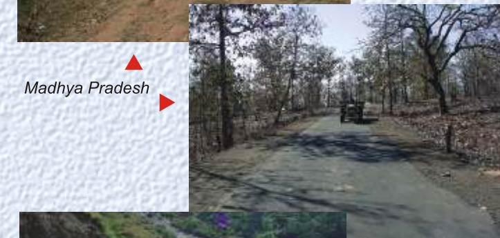
Well designed curve and super elevation
