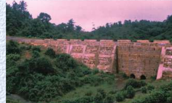
Cross Drainage & Protection Work- Meghalaya
