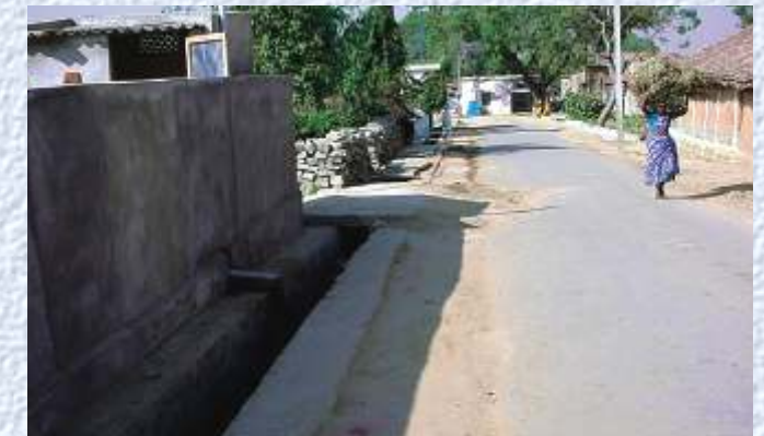
Side Drainage in built-up areas - Andhra Pradesh
