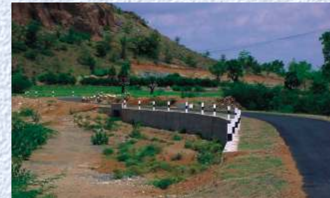
Culvert with adequate protection- Tamil Nadu
