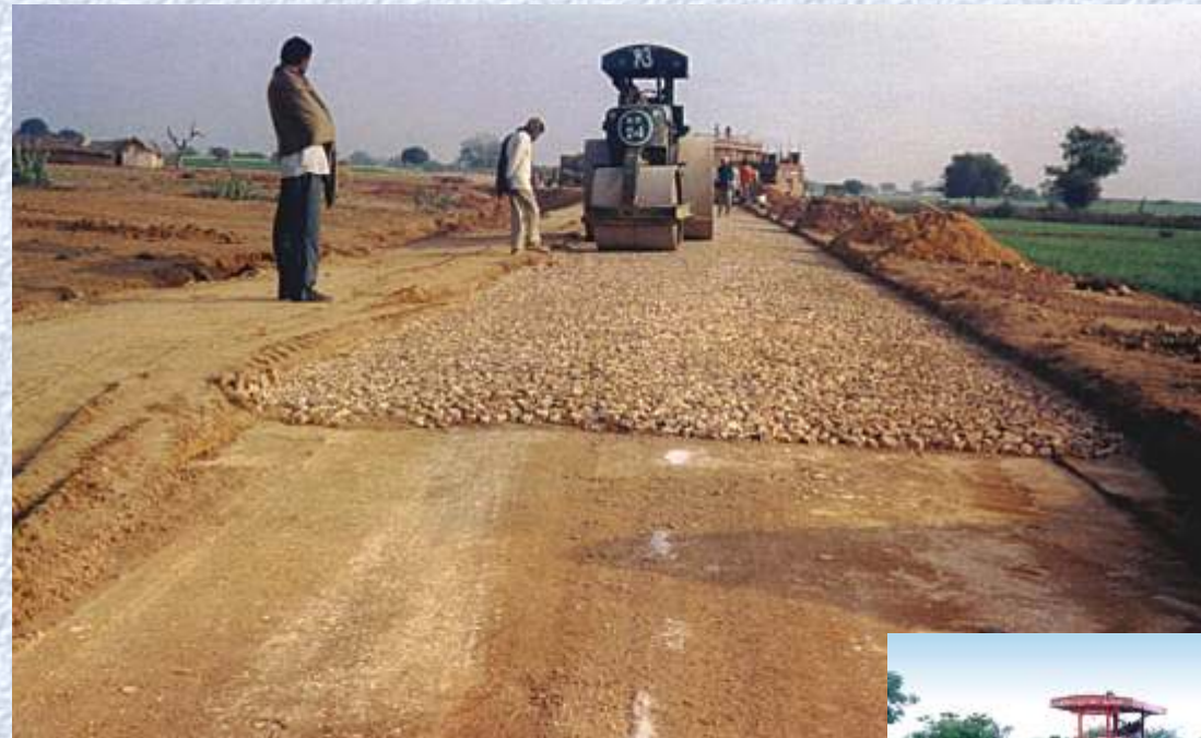
Dry Rolling of WBM in confinement - Madhya Pradesh
