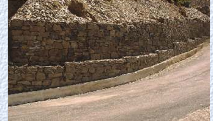
Hill Protection Work- Himachal Pradesh
