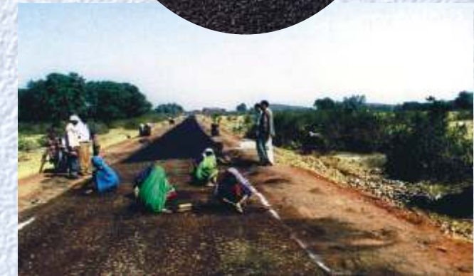
Cleaning of WBM and Laying Premix Carpet - Rajasthan
