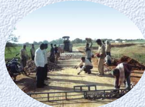
Aggregate Laying in Camber - Madhya Pradesh
