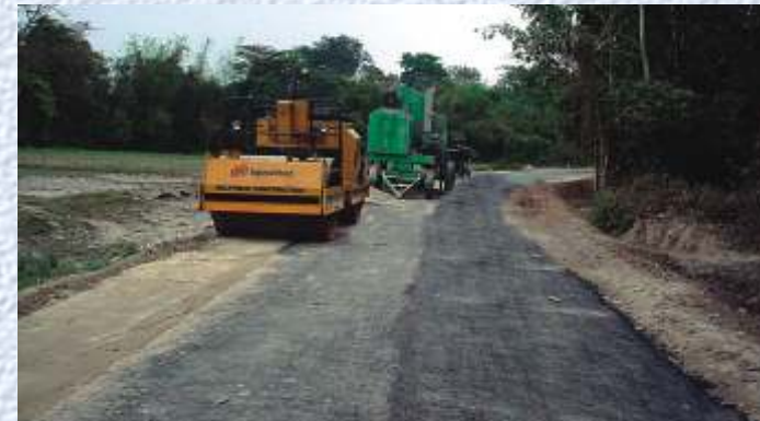
Planned Operation: Mini hot mix Plant and Roller
