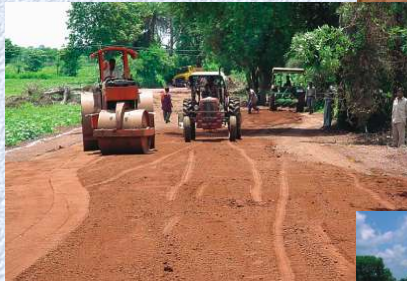
Spreading & Compacting Earth
