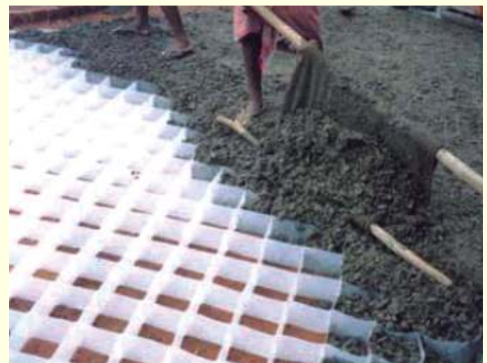
Fig.3 Placing of concrete in plastic cell
