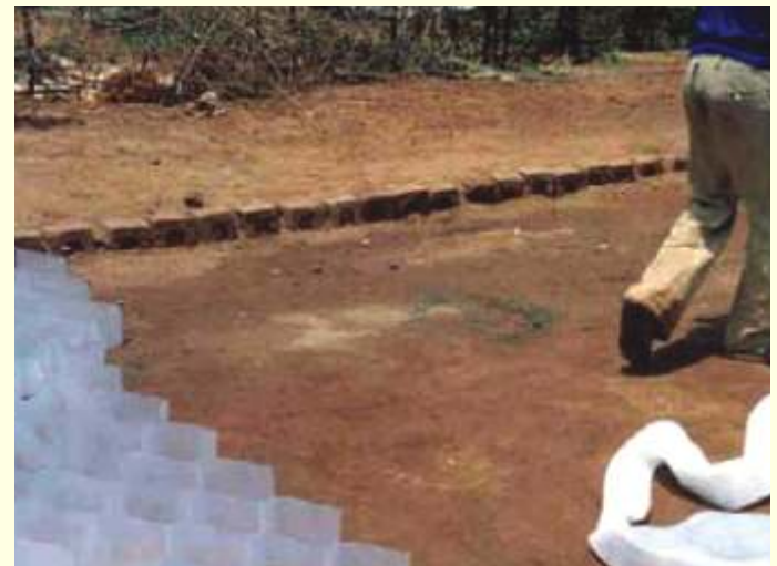
Fig 2 Formwork of plastic cell being spread
