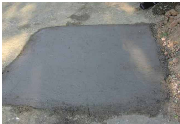
Fig.4: A view of finished surface
