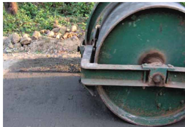
Fig.3: Rolling of cement-sand filled into cells
