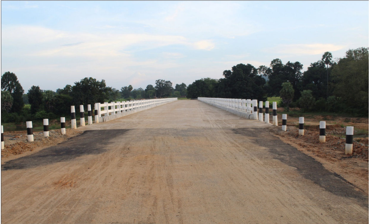
L063-PWD road to Chhatapipal road including Constriction of Bridge over Sonegarh river on PWD road to Chhatapipal ( 4 x 30.63 mtr. )under PMGSY Package No. OR-05-285/B-III.
