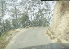
Since the road has typical hilly road geometry with series of sharp bends and steep vertical gradient and hairpin bends, speed will be automatically be less on the road. But due to non-visibility at bends with steep up or down gradient, there will always be a chance of head on collision for vehicle coming from opposite directions.
