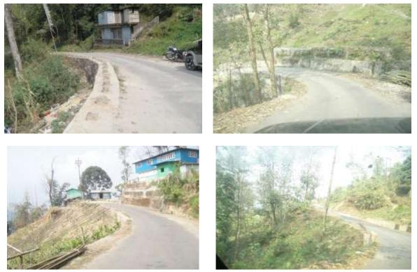
Many places on the road no wheel guard in the form of parapet wall or other was observed to protect running vehicle from overtopping on the valley side .
