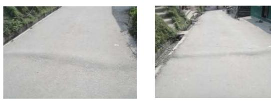
Though very few speed breakers observed on the project road as trafic calming instrument, they are found of non standard type nd not serving the purpose for which they are biult.
