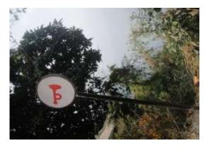
Traffic signs installed on the project road are non standard and non reflective type.
