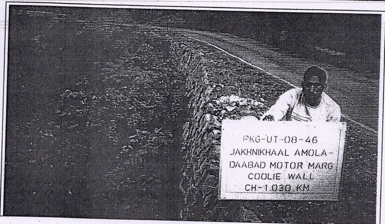
COOLIE WALL AT CHAINAGE - 1.030 KM
