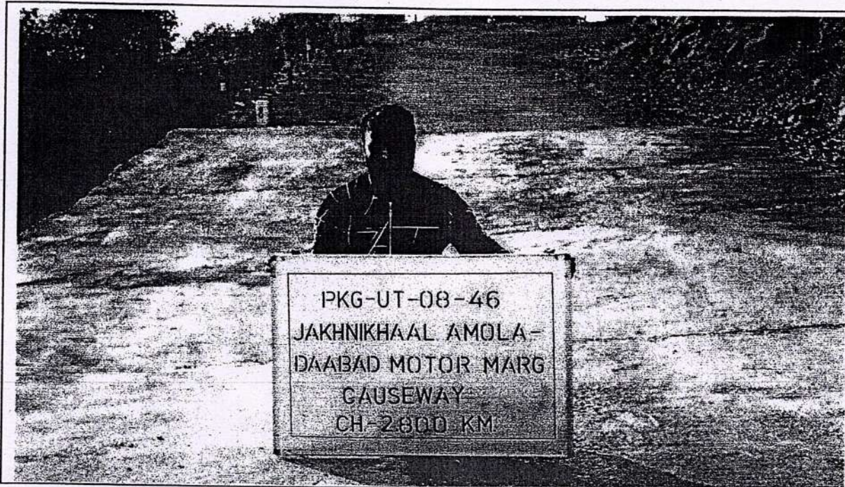
CAUSEWAY AT CHAINAGE - 2.800 KM
