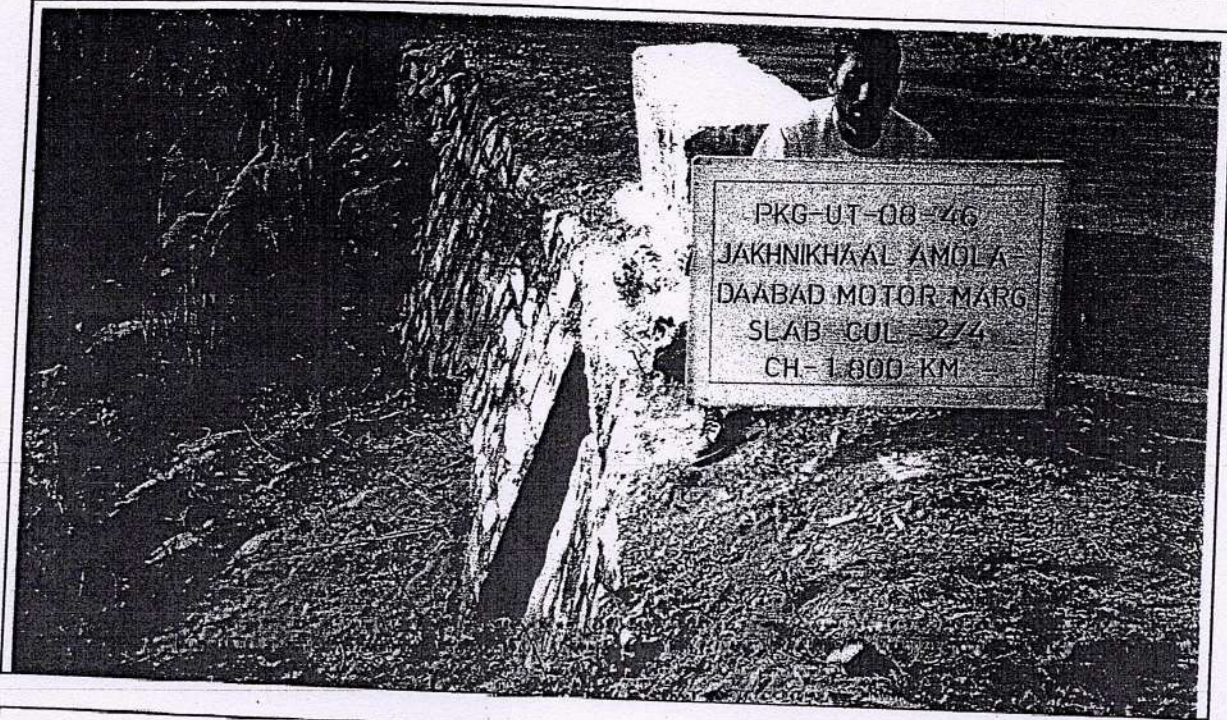
SLAB CULVERT AT CHAINAGE - 1.800 KM
