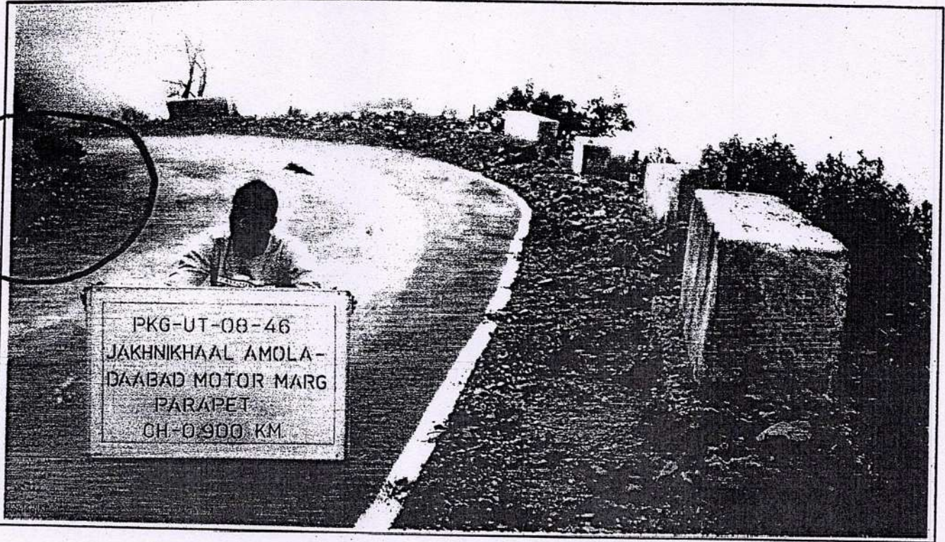
PARAPET AT CHAINAGE - 0.900 KM
