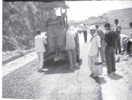
Photo 8: Compaction of cold mix
