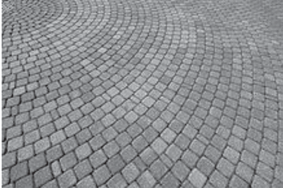
Concrete paver blocks in a circular pattern
