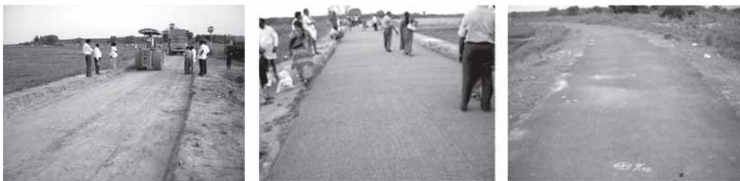
Fig.6. Finished subgrade
