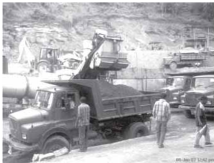
Photo 1: Preparation of Cold Mix for BM
