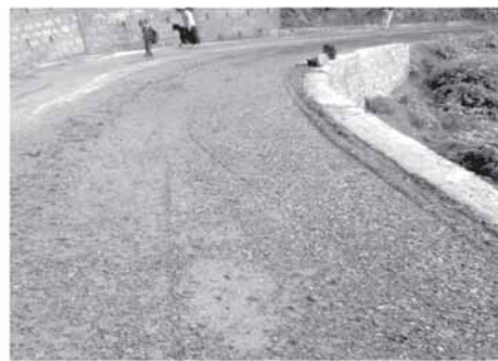
Photo 2: Finished BM on By-pass by Hot Mix Plant Aizawl
