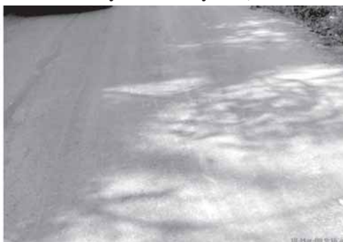
Photo 10 : Good Performance of MSS after One Year in Aizawl
