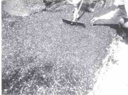
Photo 7: Spreading cold mix
