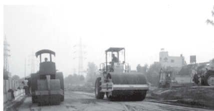
Construction of Sarita Vihar Fly over , New Delhi
