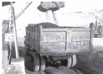
Photo 6: Discharge of Cold Mix
