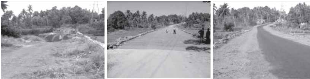
Fig.3. Before construction Fig.4. During construction Fig.5. After construction
