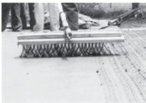
Texturing of Concrete for anti-skid finish
