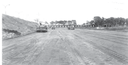
Approach Road Embankment, Nizamuddin
