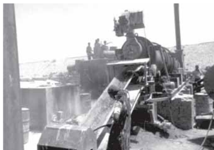
Photo 5: Adding water in Aggregates
