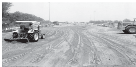
Construction of Panjabi Bagh Fly over , New Delhi
