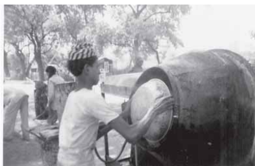
Photo 1: Charging aggregates into mixer
