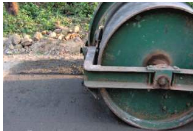
Fig.3: Rolling of cement-sand filled into cells
