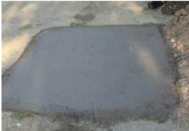
Fig.4: A view of finished surface
