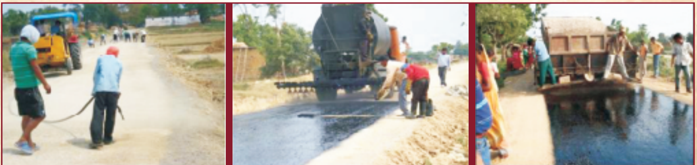
FIGURE 2. Otta Seal Laying Process cleaning, bitumen spray and chips spreading.
