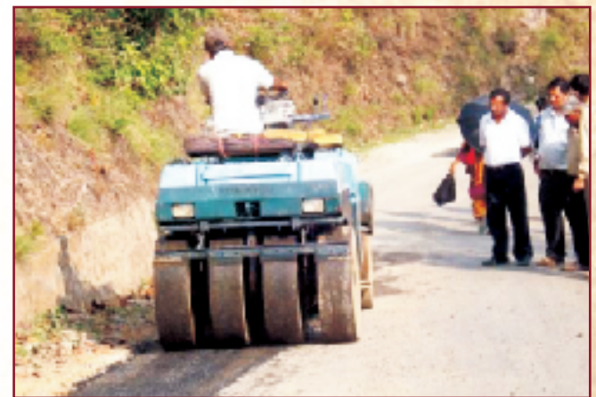
FIGURE 6. Otta Seal maintenance
